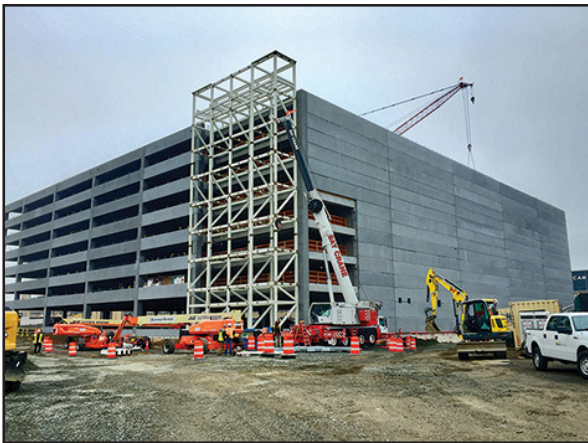
Construction Inspection West Parking Garage - LaGuardia (LGA) Redevelopment Program (PANYNJ)
