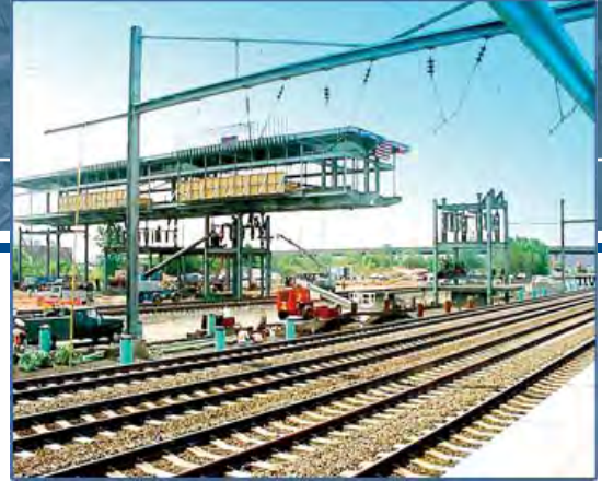
Construction Management Services for Northeast Corridor-Newark Liberty International Airport AirTrain Extension [NJ TRANSIT]
