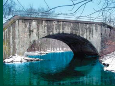
Inspection, Load Rating and Design of Port Jervis Line Undergrade Bridges - MTA / MNRR
