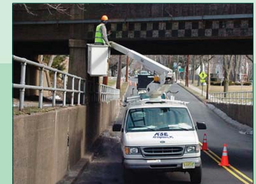
Indepth Inspection and Load Rating of 59 Undergrade Bridges - NJ Transit
