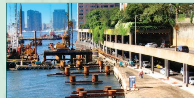
Construction Inspection for the FDR Drive Southbound Roadway Reconstruction and Outboard Roadway Reconstruction - NYSDOT
