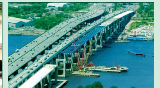
Prime Construction Engineering Consultant for New Route 9 Southbound Bridge Over Raritan River - NJDOT
