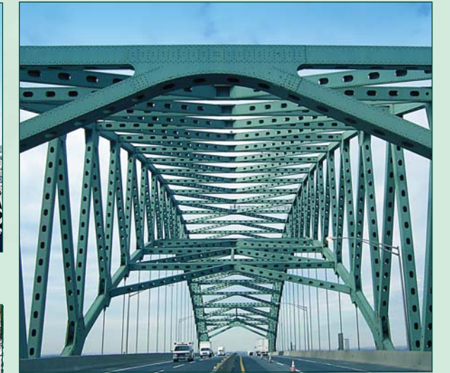
Structural Inspection & Design of Delaware River Bridge Deck Reconstruction - NJ Turnpike
