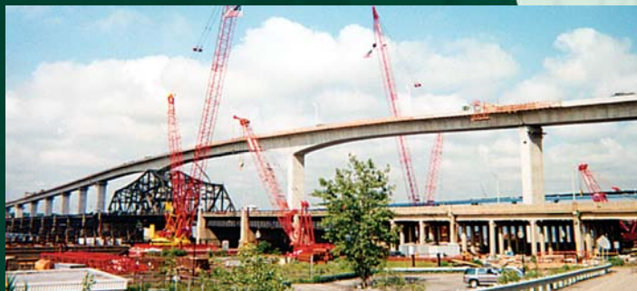
Construction Inspection Services for the Victory Bridge / Route 35 Replacement over the Raritan River - NJDOT
