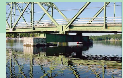
Underwater Inspection of over 150 Structures in Regions 1, 2, 7, 8, & 9 - NYSDOT
