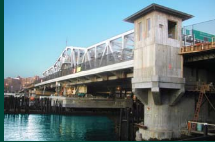
Construction Inspection for the Replacement of the Third Avenue Swing Bridge Over the Harlem River - NYCDOT
