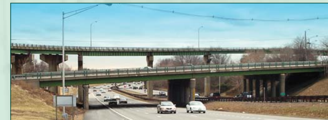
NBIS Inspection of 85 Bridges MP 94.8 to 168 - NJTA / GSP DIV
