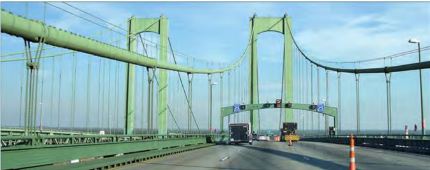
NBIS Inspection of Delaware River Memorial Bridges [DRBA]
