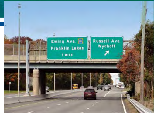
Inspection of 127 Overhead & Cantilever Sign Structures [NJDOT]
