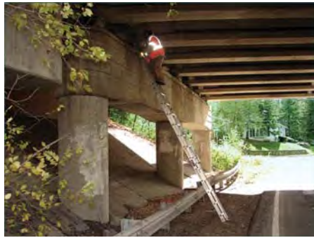
NBIS Inspection of 42 State Bridges [NJDOT]
