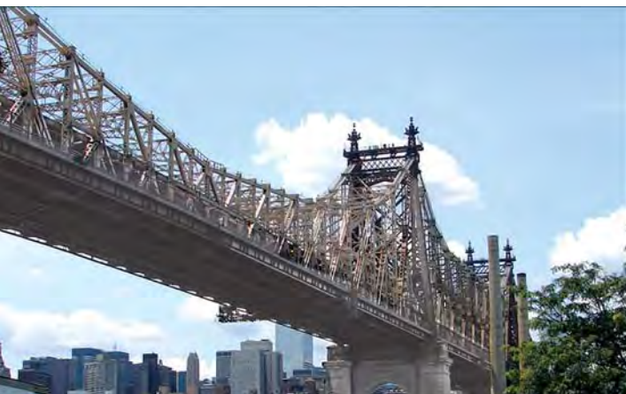
Biennial & Interim Inspection of the Queensboro Bridge [NYSDOT]
