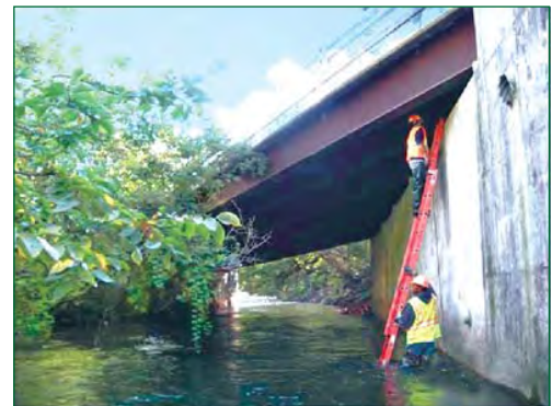
Biennial & Interim Inspection of 900 Region 2 Bridges [NYSDOT]
