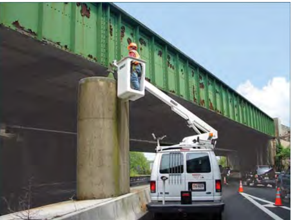
FCM Inspection of Garden State Parkway Bridges over Rt. 166 [NJTA]
