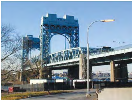
Biennial Bridge Inspection & Design of Miscellaneous Structural Repairs at the Robert F. Kennedy Bridge [TBTA]
