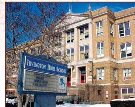
Construction Management of Irvington Township Schools - NJSCC
