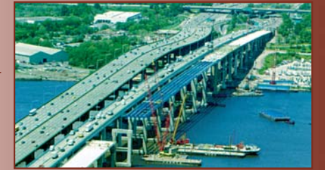
Prime Construction Engineering Consultant for New Route 9 Southbound Bridge Over Raritan River - NJDOT
