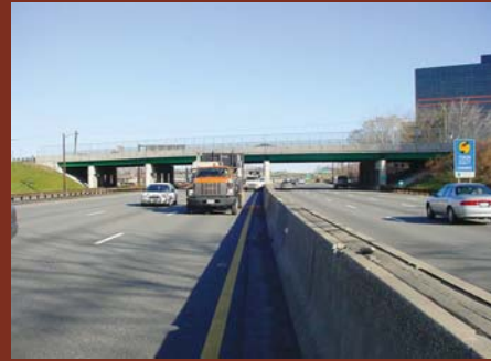
Construction Inspection for Various Reconstruction, Rehabilitation and Repair Projects Systemwide - NJTA
