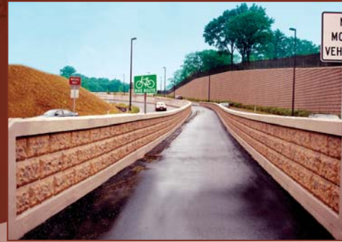
Construction Engineering, Administration and Inspection for Route 18 Extension / Rutgers Improvements - NJDOT 2006 ACECNY Platinum Award Winner
