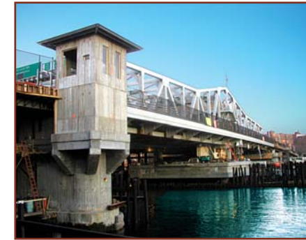
Construction Inspection for the Replacement of the Third Avenue Swing Bridge over the Harlem River - NYCDOT
