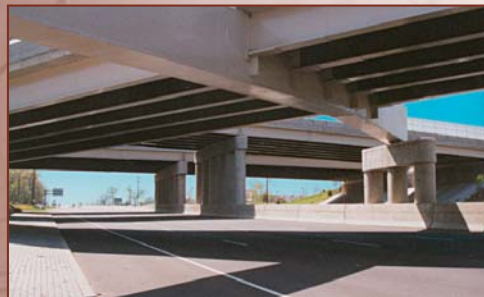
Construction Inspection for Route 1 & 130 / Georges Road Circle Elimination and Intersection Reconstruction - NJDOT
