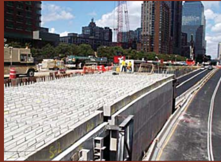
Construction Inspection for Route 9A Promenade South - NYSDOT
