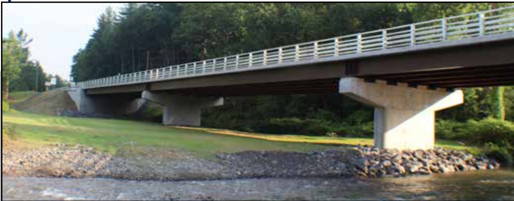
◀ Design-Build, Region 8 Bundled Bridges, Replacement of Two Bridges, Route 28 Bridge & Route 209 Bridge, Ulster County, NY NY State Department of Transportation (NYSDOT)
