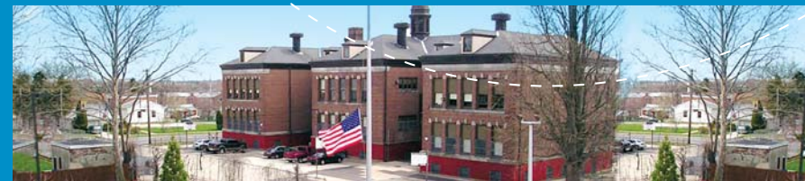
Civil Design Services for Renovations Penrose Elementary School & Motivation High School Philadelphia, PA
