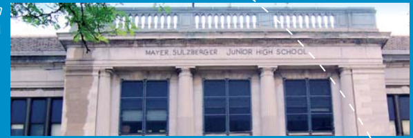
Facade Rehabilitation Mayer Sulzberger Middle School - Philadelphia, PA
