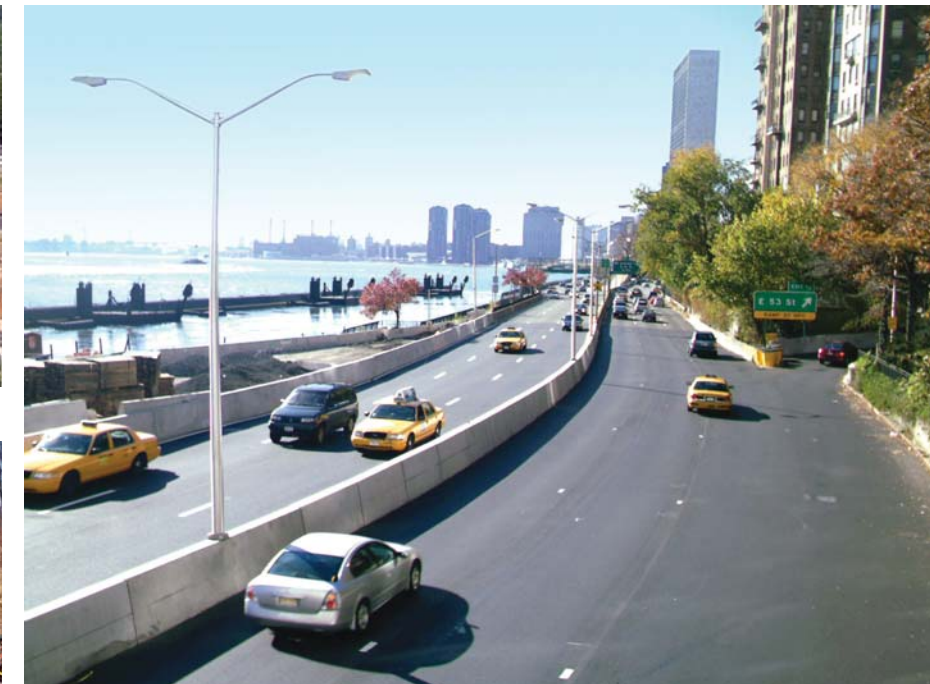
Construction Inspection for FDR Drive SB (E. 56th to E. 64th St.) Reconstruction - NYSDOT
