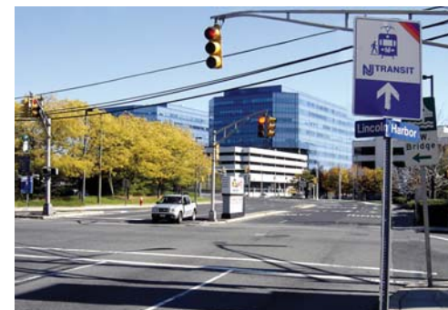
Traffic signal Improvements for 10 Intersections - Hudson County NJ
