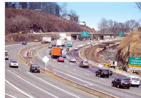
Construction Inspection Services for Westchester Expressway - NYSDOT
