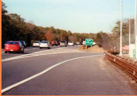
Garden State Parkway Interchange 77- NJTA
