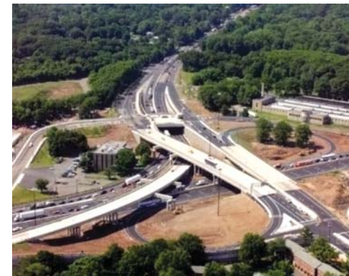
Construction Inspection for Route 1 & 130 - NJDOT
