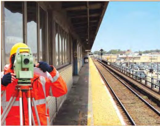
Shea Stadium Platform Topographic Survey [MTA-LIRR]
