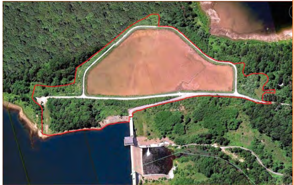
Charlotteburg Reservoir Sludge Lagoon Topographic Survey [City of Newark]
