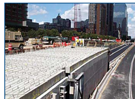
Construction Inspection Services for Route 9A Promenade South - NYSDOT
