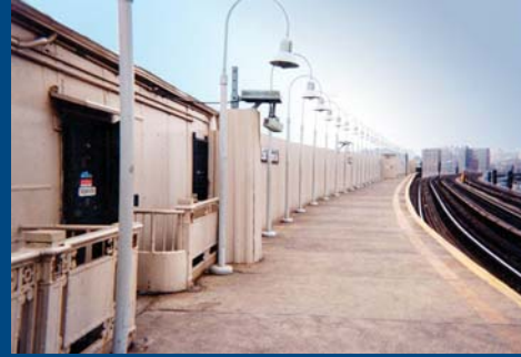
Civil Engineering - Sixteen Stations on White Plains Rd. Bronx - MTA / NYC Transit
