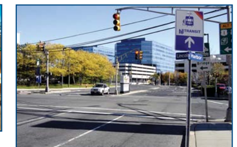
Traffic signal Improvments for 10 Intersections - Hudson County NJ
