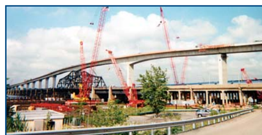
Victory Bridge / Route 35 Pre-Cast Segmental Continuous Span Bridge - NJDOT
