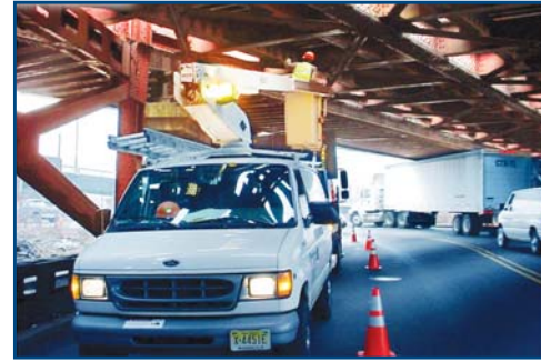
Undergrade Bridge Inspection - Morristown Line - NJ Transit
