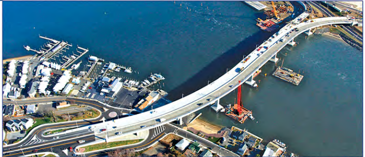
Construction Inspection Services for Route 36 Highlands Bridge over Shrewsbury River [NJDOT]
