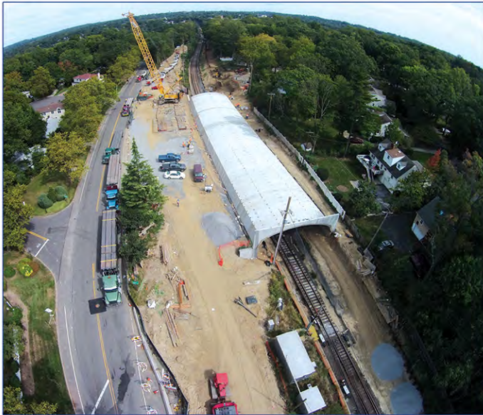
Design-Build Services for Colonial Road Improvements and Pocket Track Extension [LIRR]
