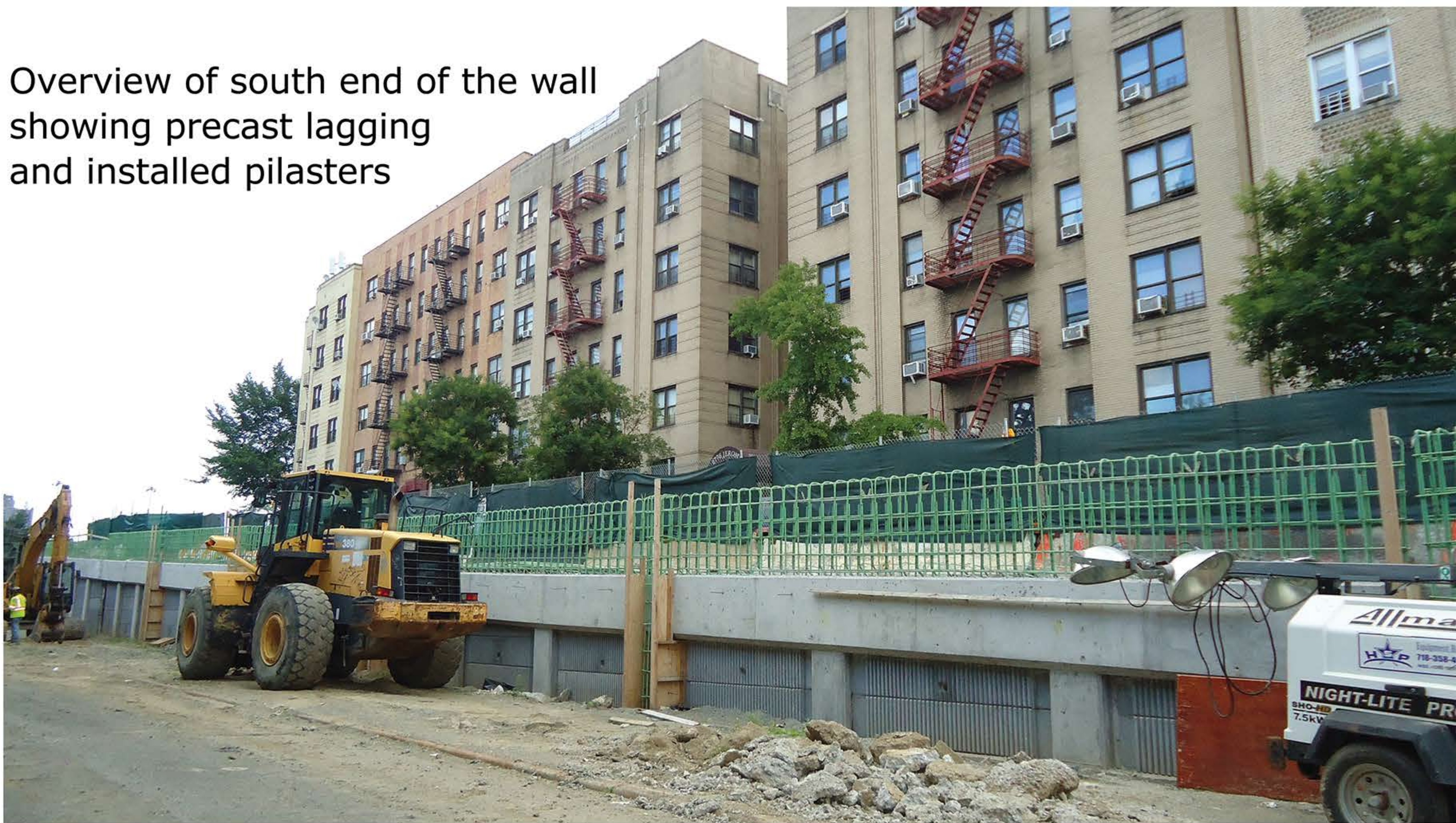
Constructing the south end of the parapet wall with the rebar work in progress
